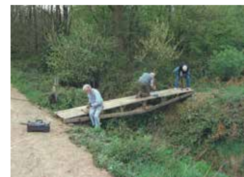
A temporarily inverted bridge being prepared on site.
