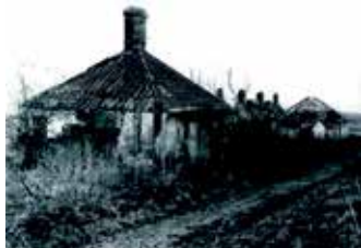
High Park Farm Cottages 3 & 4 Photos 1945
