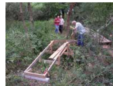
A temporarily inverted bridge being prepared on site.
